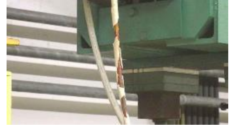
Cabling status inspection
