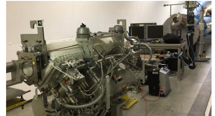
Remote Vacuum Leak detection
