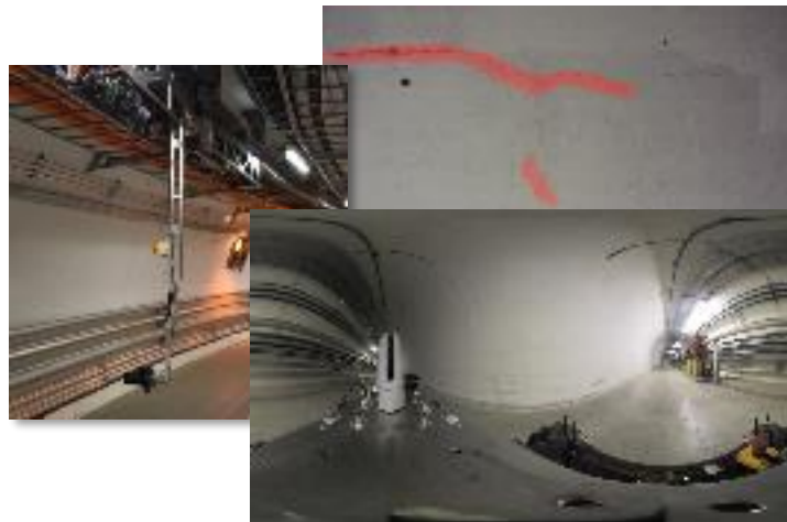
Tunnel structure monitoring
