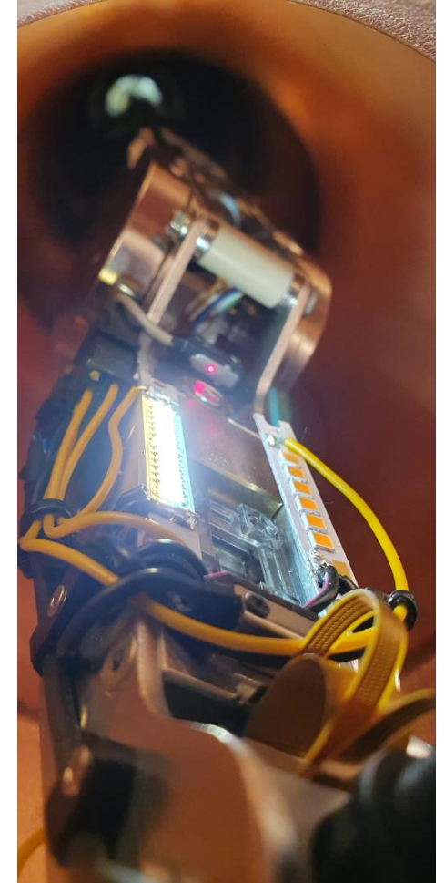
Robotic arm inside the cavity
